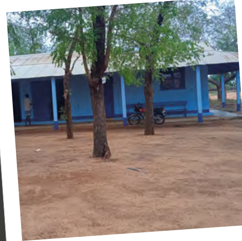
Extending and rehabilitating DFM's local office at SALFA Ejeda.
